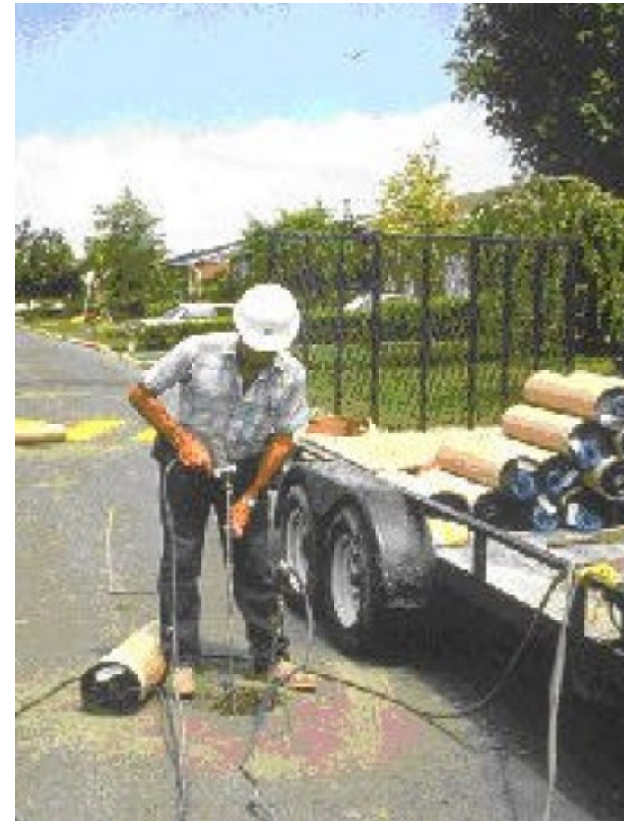
Attaching anode wire to pipe using electrical resistance welding
