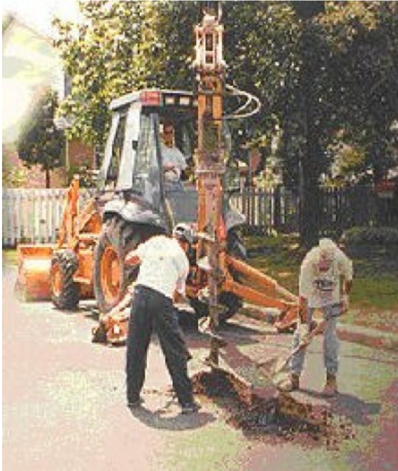
Using auger to drill anode holes
