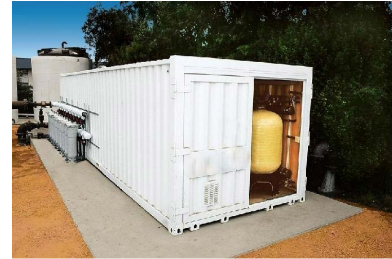
1,000-GPM Nitrate Removal System - California
